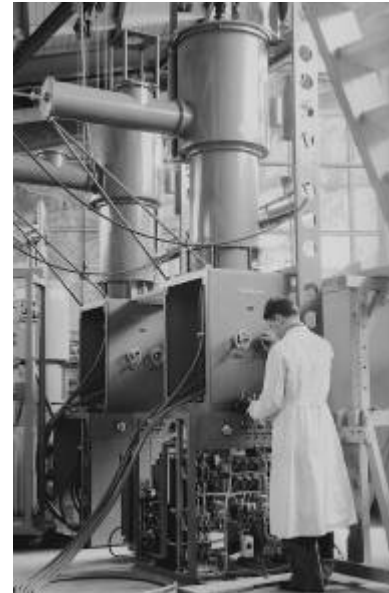
200 MHz triode amplifier (CERN Linac3)
