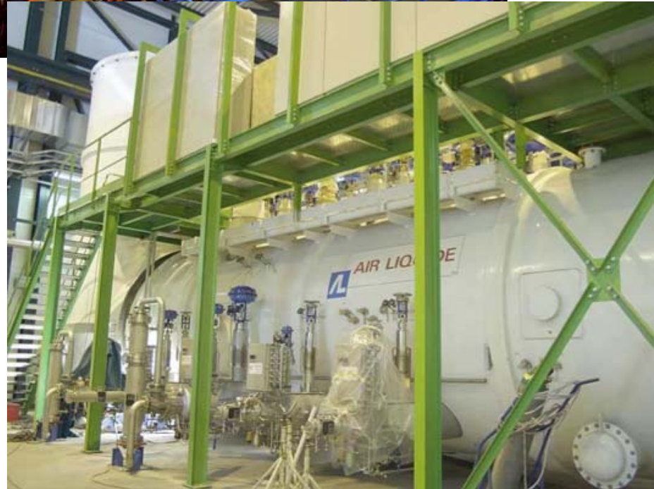
LHC refrigerators: \approx 140 \text{ kW @ } 4.2 \text{ K}
