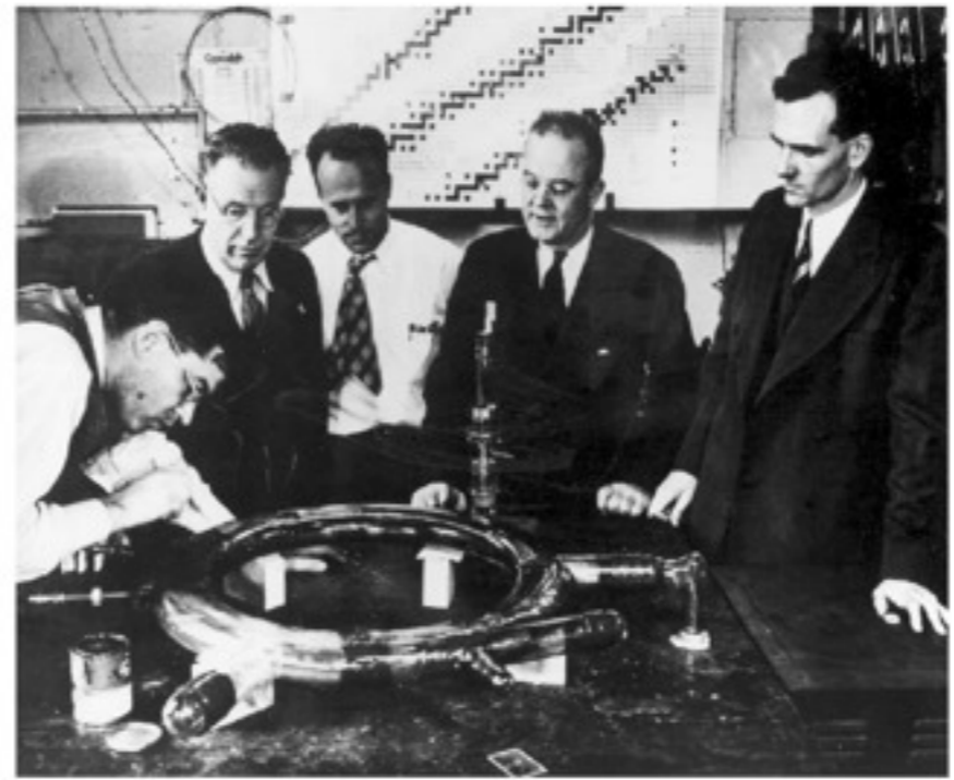
Figure 5 The General Electric team (from left to right, Langmuir, Elder, Gurewitsch, Charlton and Pollock) looking at the vacuum chamber of the 70 MeV synchrotron – the world's second synchrotron.
