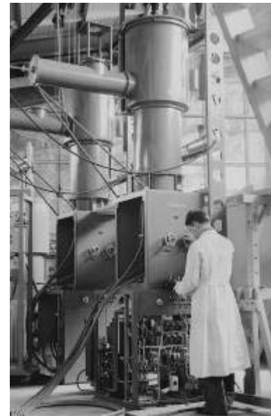
200 MHz triode amplifier (CERN Linac3)
