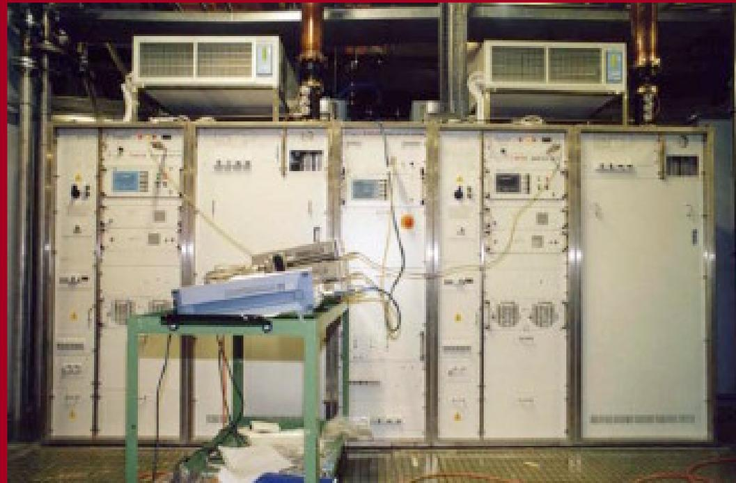
New 150 kW CW transmitter for the ELETTRA
