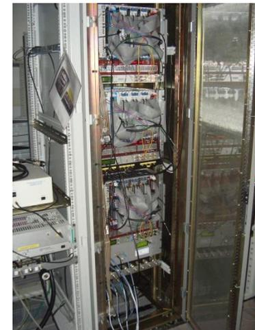
↘ **CESR** transverse and longitudinal feedbacks: they employ VME digital processing boards equipped with ADC, DAC, FIFOs and PLDs
