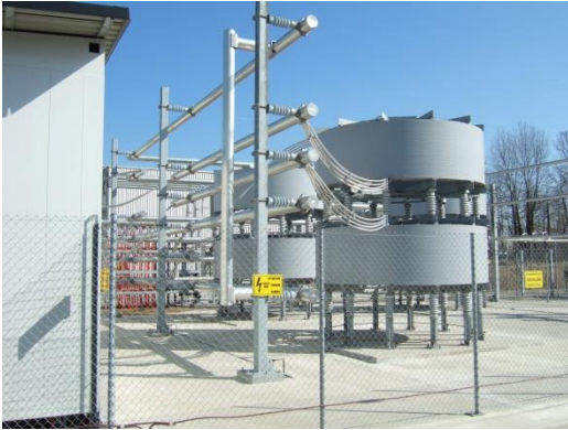
TCR reactors (50 Mvar / ph)
