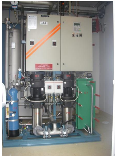
Cooling plant for thyristor valve
