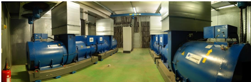
Two twin rotablocs (4 accumulators and 4 alternators in one cell)
