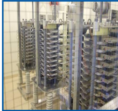
Thyristor valve 18 kV, 2800 A
