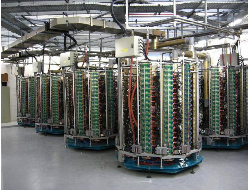
45 kW per tower (2004 and 2007)
