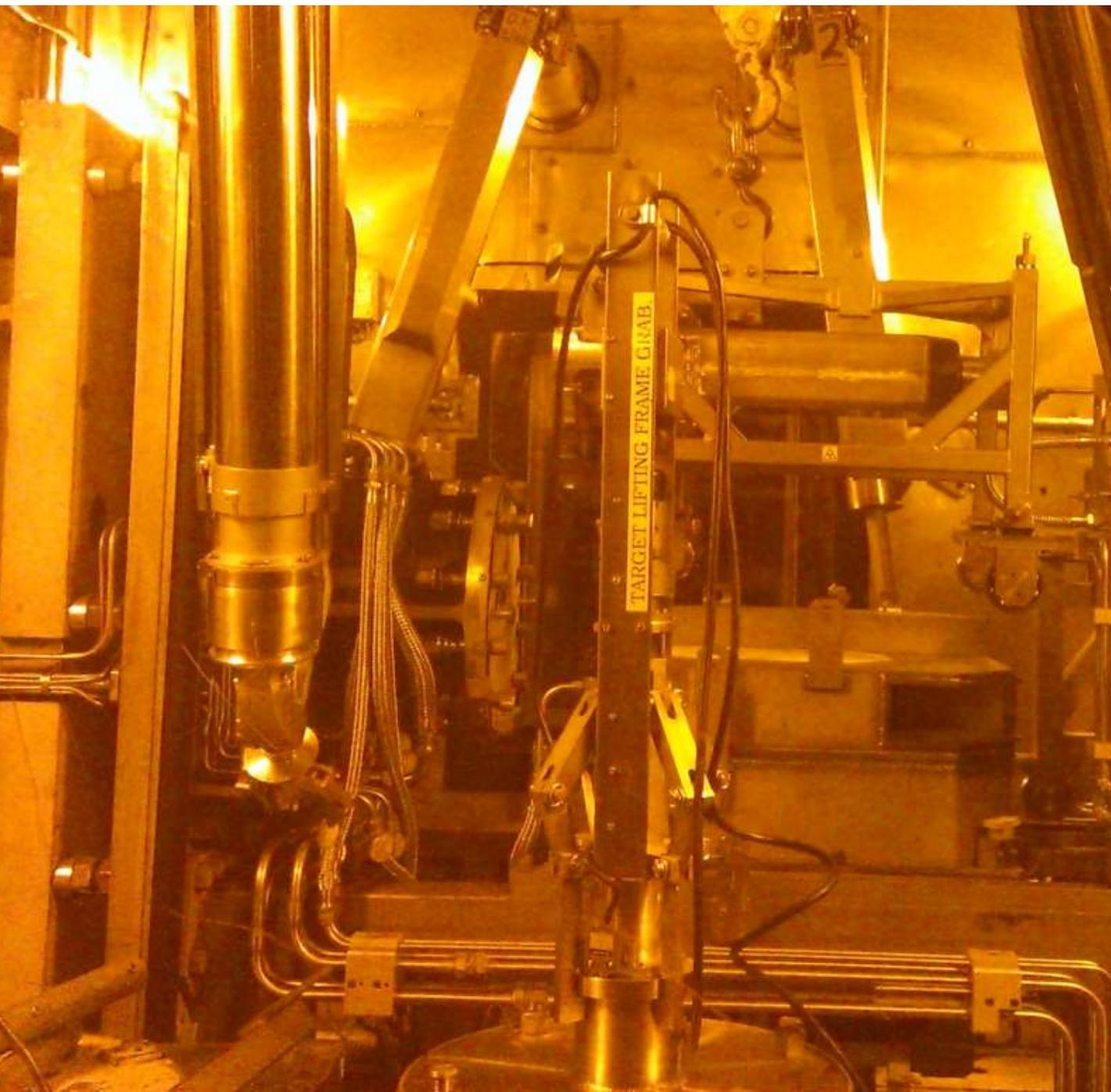
The target has been disconnected and is being lifted away from its working position
