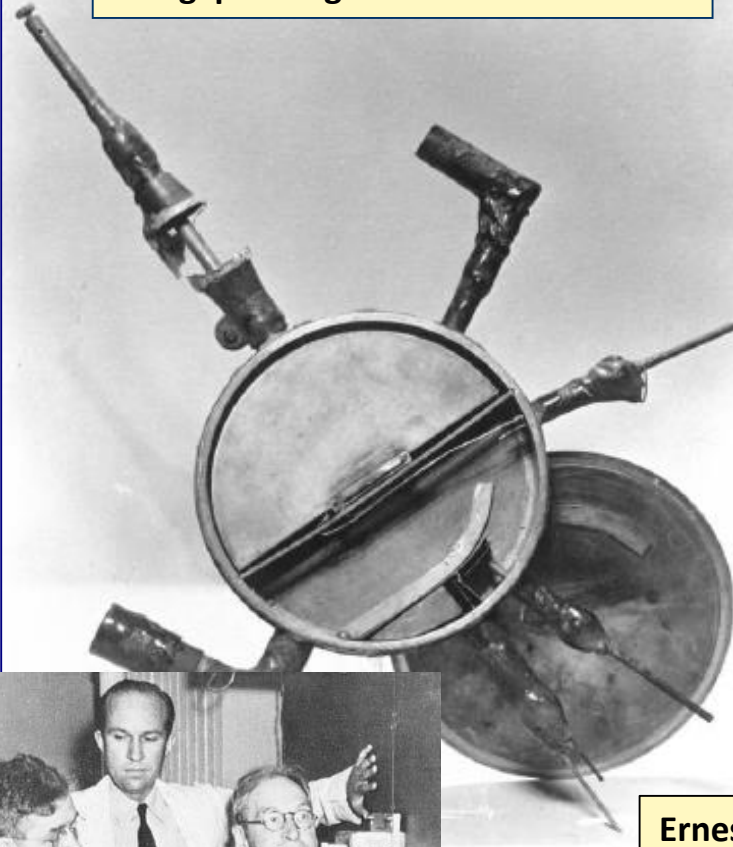
first cyclotron: 1931, Berkeley 1kV gap-voltage 80keV Protons
