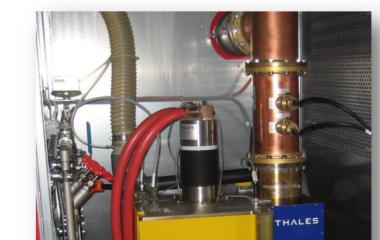
IOT's are the main component of the transmitter. They provide 80kW of RF power in CW with a maximum efficiency of 70%.
