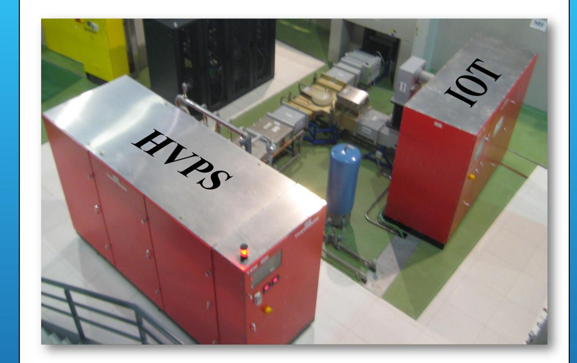
The HVPS provides up to -38kV 4A to the IOT. It uses 60 switching modules, up to 3 can fail at the same time without affecting operation.
