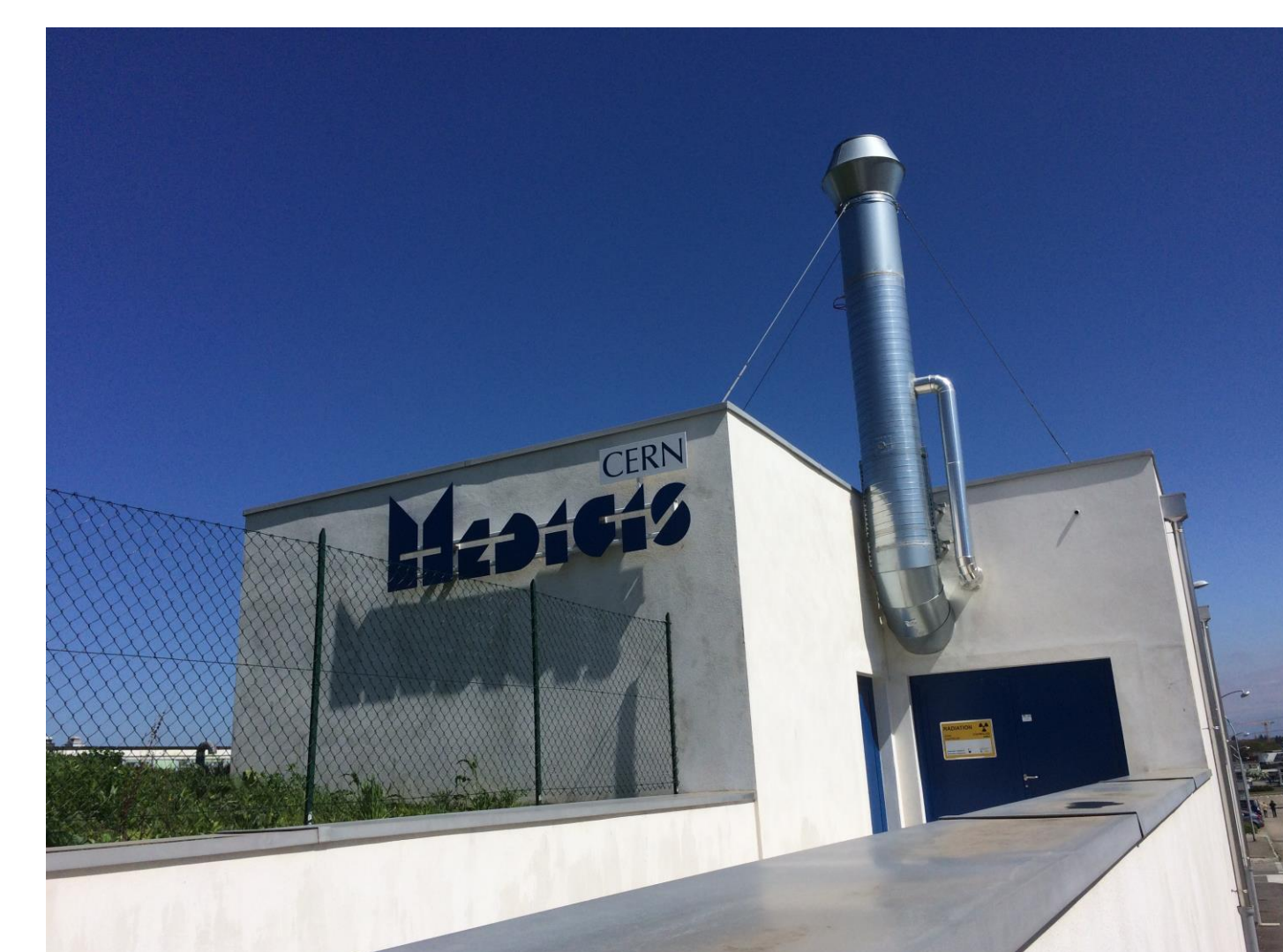
The MEDICIS facility under construction at CERN.
