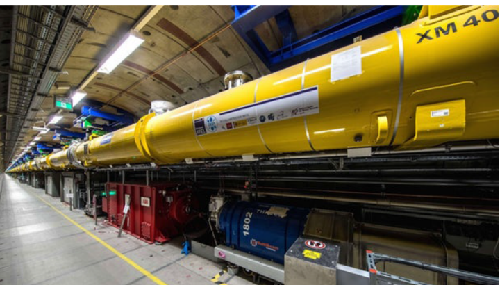
XFEL in operation since Dec 2016
