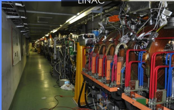
DRIVE BEAM LINAC
