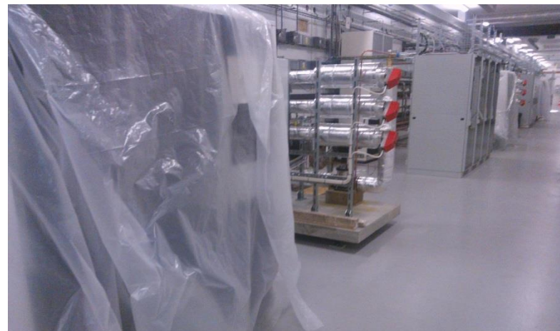
Modulators and SHG partially installed
