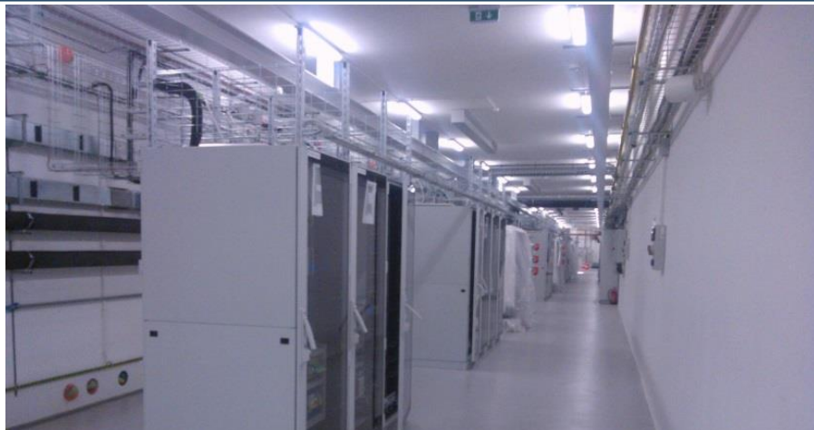
Racks with equipments installed
