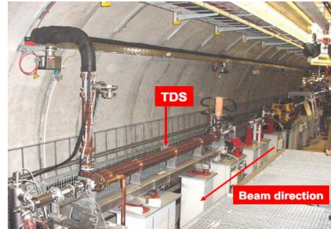
TW RF deflector @ FLASH
