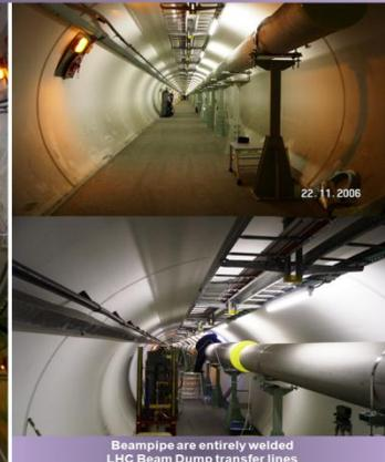
Beampipe are entirely welded LHC Beam Dump transfer lines
