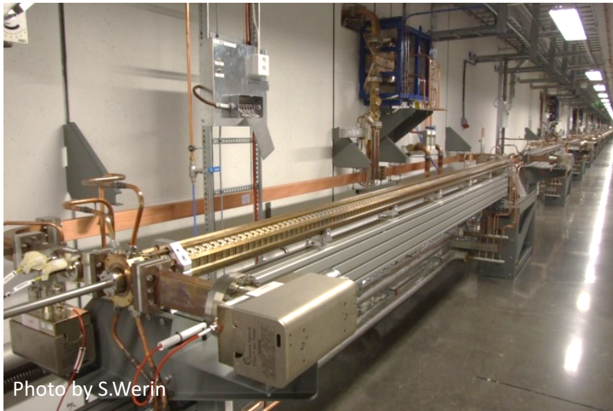
MAX IV Full Energy Injector LINAC
