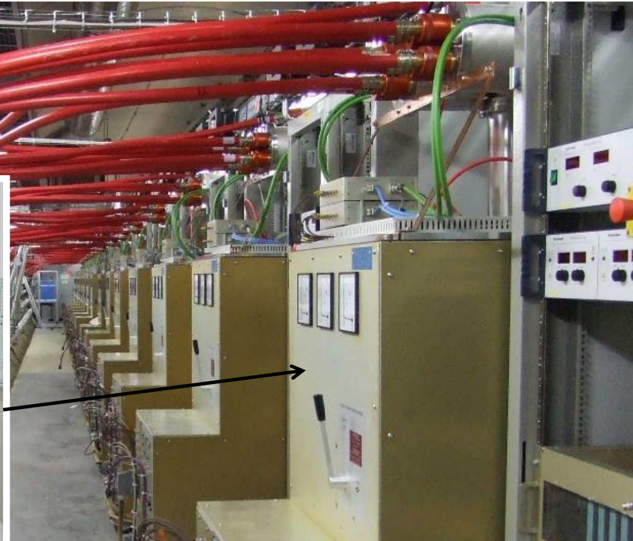
Fast High Current Thyristor stack with trigger transformer
