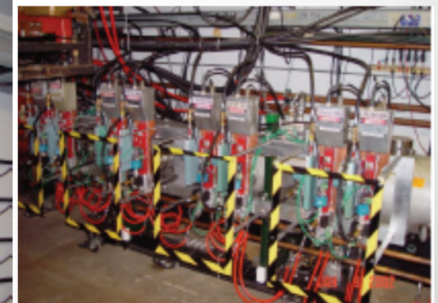
power amplifiers (TWTs)
