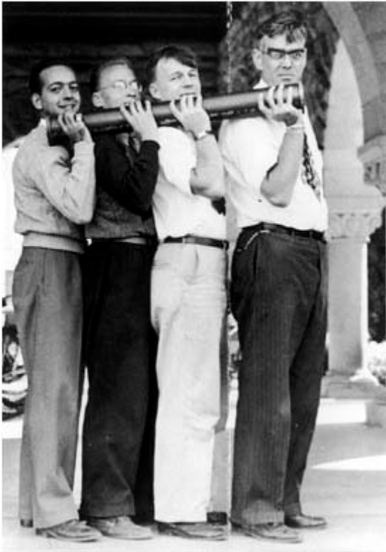
William Hansen (right) and colleagues with a section of the first electron linear accelerator that operated at Stanford University in 1947. It was 3.6 meters long and could accelerate electrons to 6 MeV.
