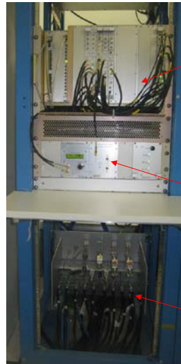
Cavity Controller VME crate
