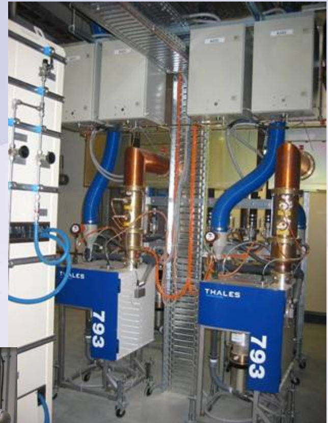
3 x IOT-based 300 kW amplifiers
