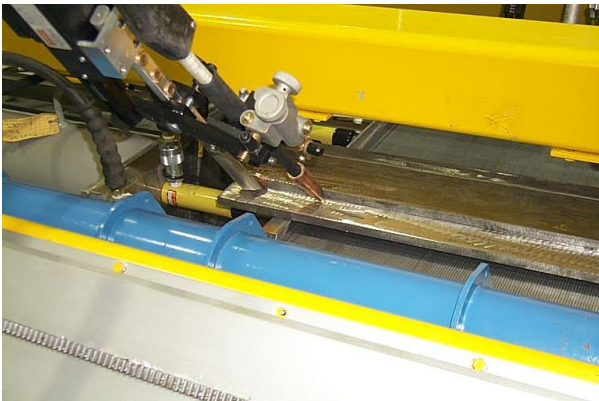
Welding the structural plates
