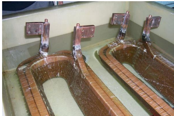
coil electrical test (under water !)
