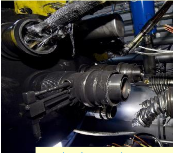
Arcing in the interconnection
