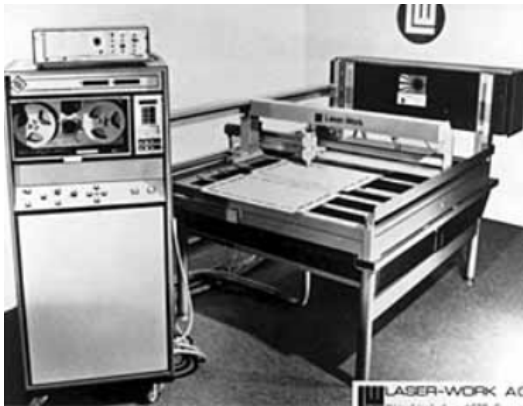
First 2 axis laser cutting machine (1975, Laser - Work AG, Switzerland)
