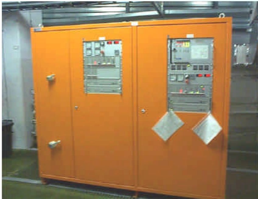
Elettra – Transfer Line Dipole Power Supplies: 2 PS (200 V / 1080 A, 12p-bridge & 60 V / 1080 A, 6p-bridge) in one cabinet.
