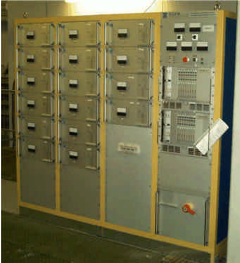
Elettra – Storage Ring Correctors Power Supplies Cabinet.
