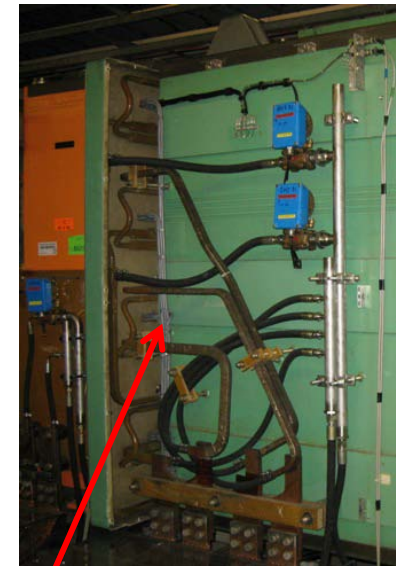
Installed Booster Dipole
