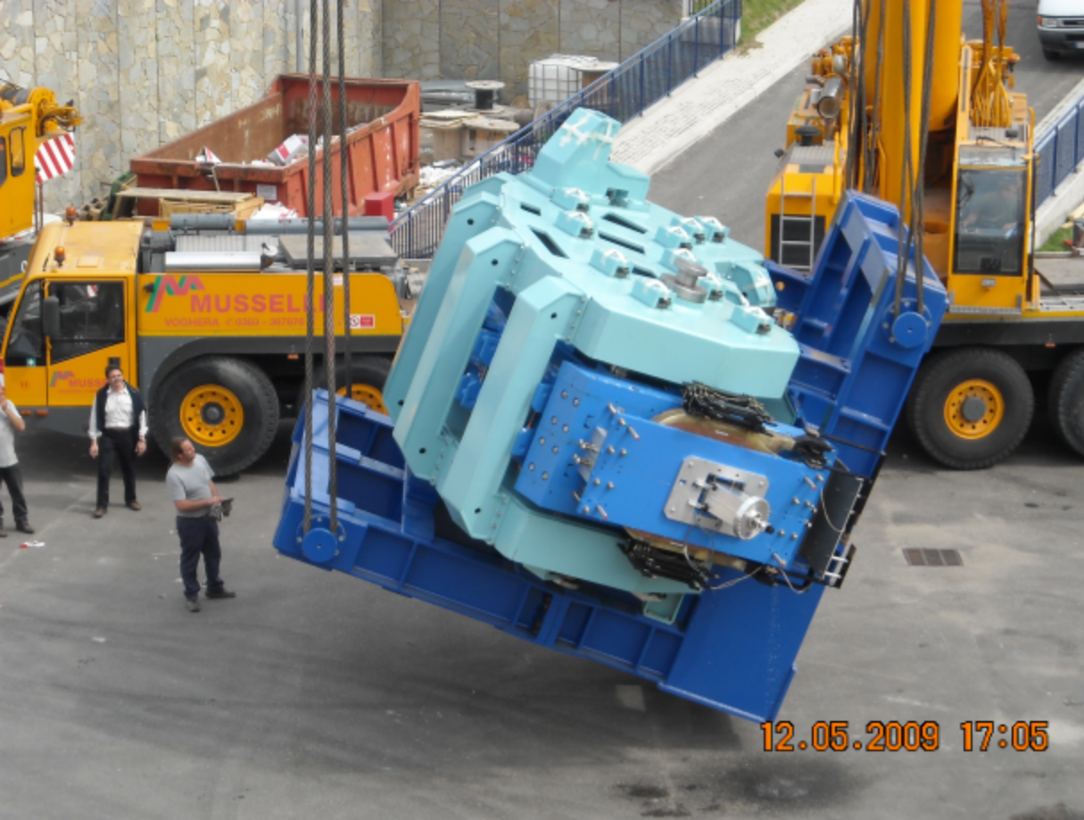
The CNAO 90° magnet during installation in the vertical line. The size is the same as for a gantry final magnet.
