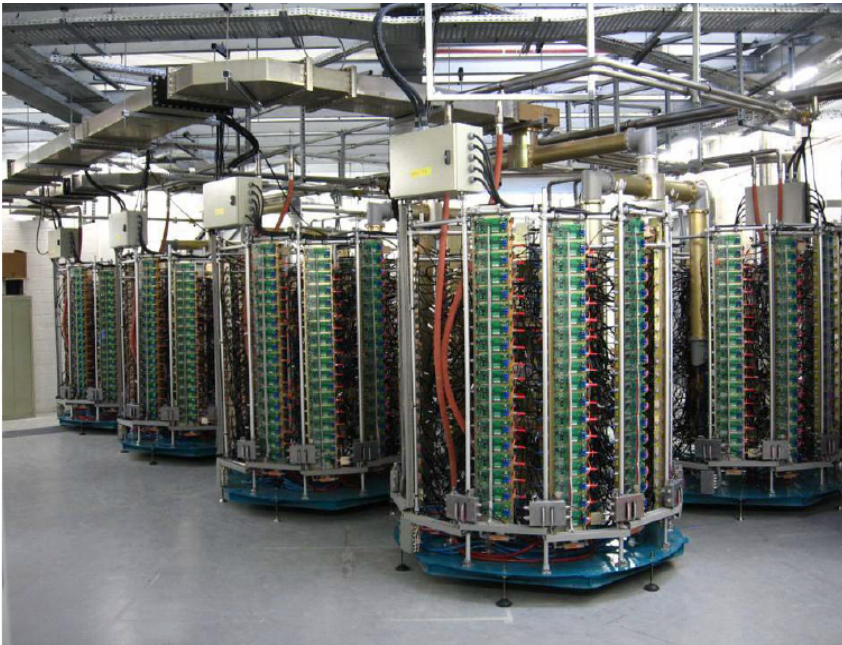
SOLEIL 45 kW @ 352 MHz solid state amplifier towers (2004 & 2007)
