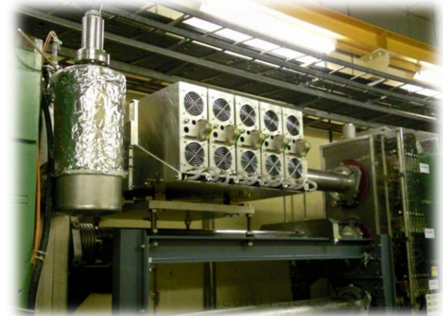
Prototype system installed in ring 4 of CERN PSB
