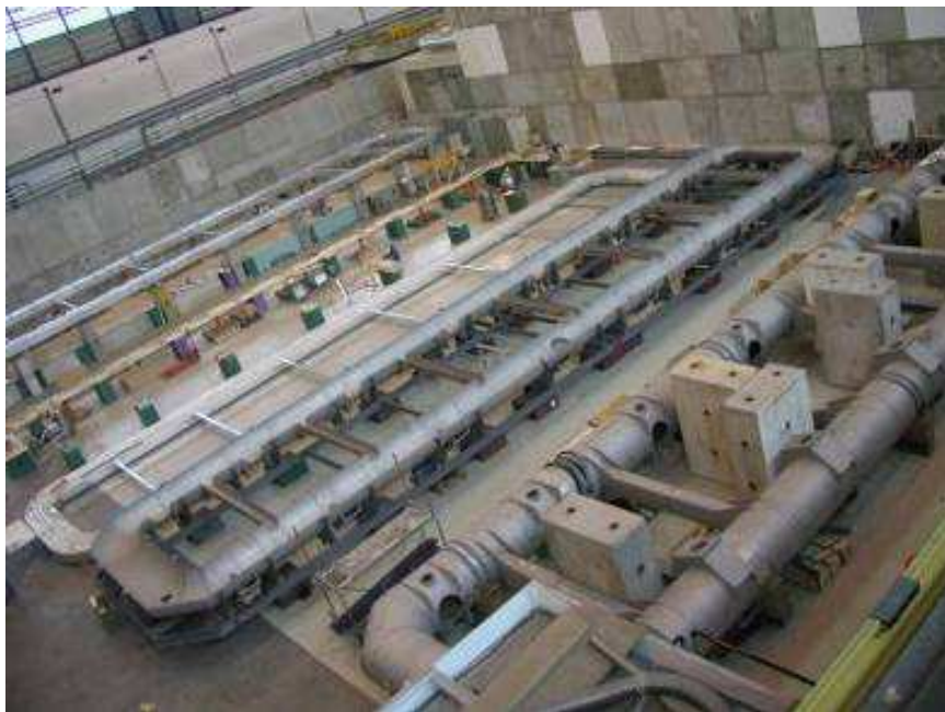
Cryostatting at CERN
