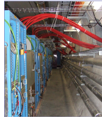
Generators nearby in gallery next to LHC tunnel
