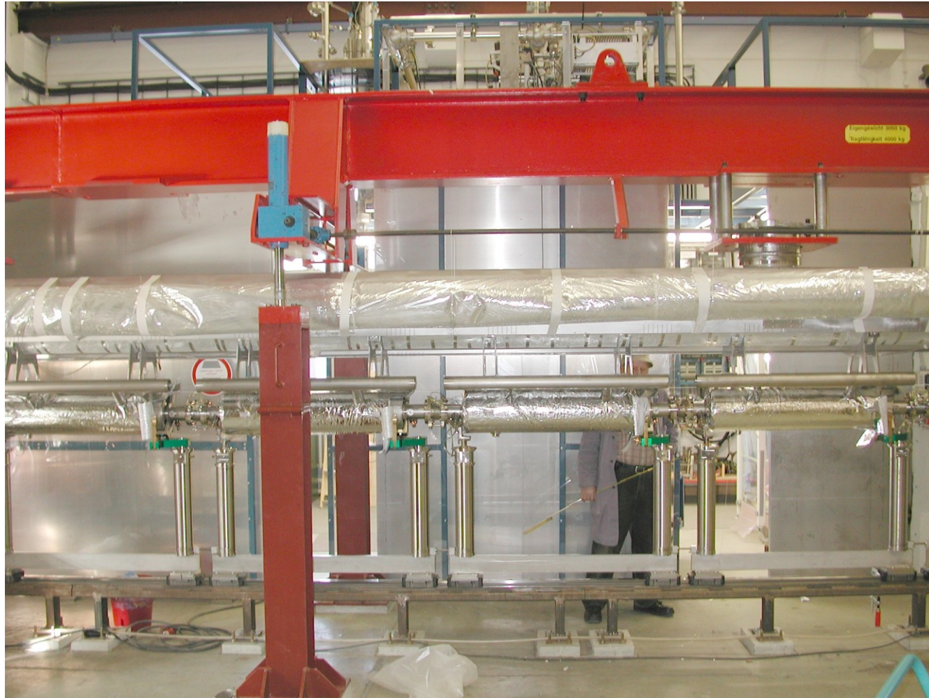
String in the assembly area
